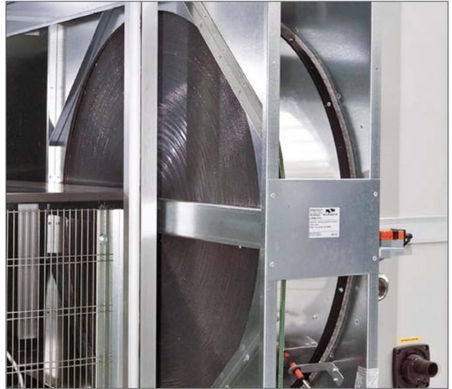
ROTARY HEAT WHEEL EXCHANGER
