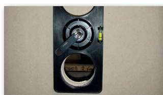
4 Attach the drilling template with the tensioner.
