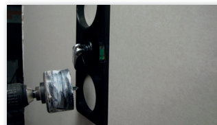
3 Then drill through the existing hole inserts.
