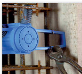
5 Simply bind to the steel reinforcement. Concrete cover to 40 mm.
