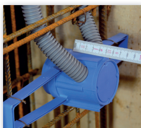
6 The assembly of the upturned wing concrete socket box also allows concrete coverage to 60 mm.
