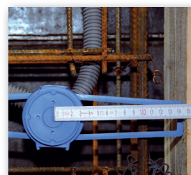
4 Allow the wings simply to cue up at the door formwork until the socket box centre (15 cm in length).
