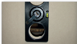
2 Precise alignment using the integrated spirit level.
