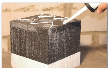
4 Apply TIE-hybrid adhesive in thin, bead form (5-6 mm).
