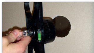
1 Drilling of the centre hole.
