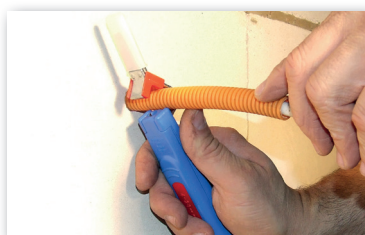
2 Cut conduit flush with the wall.
