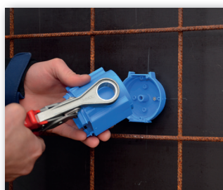
2 Punch out pipe or cable entry with the punch pliers.
