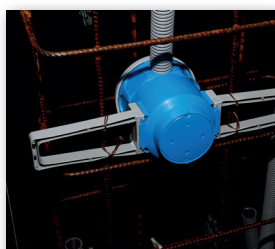
5 Assembly as electronics electronic large socket box with wings.
