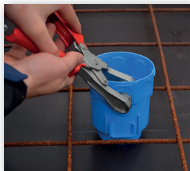
1 Punch hole out using punch pliers.
